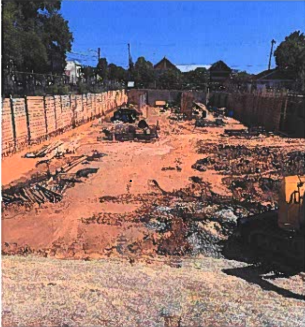
Figure 1 July 17, 2019; Looking north - excavation of footings & forming of B Line Wall
