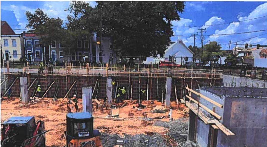
Figure 2 August 8, 2019; Looking west - forming of B Line Wall
