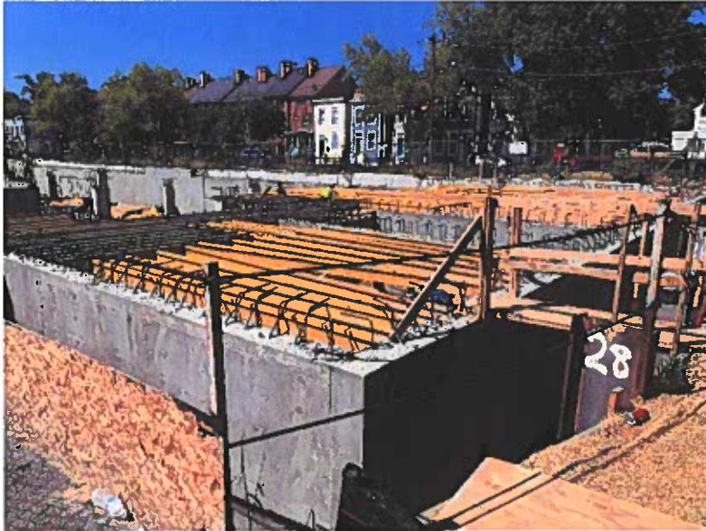
Figure 1 September 3, 2019; Looking south at cast in place deck shoring
