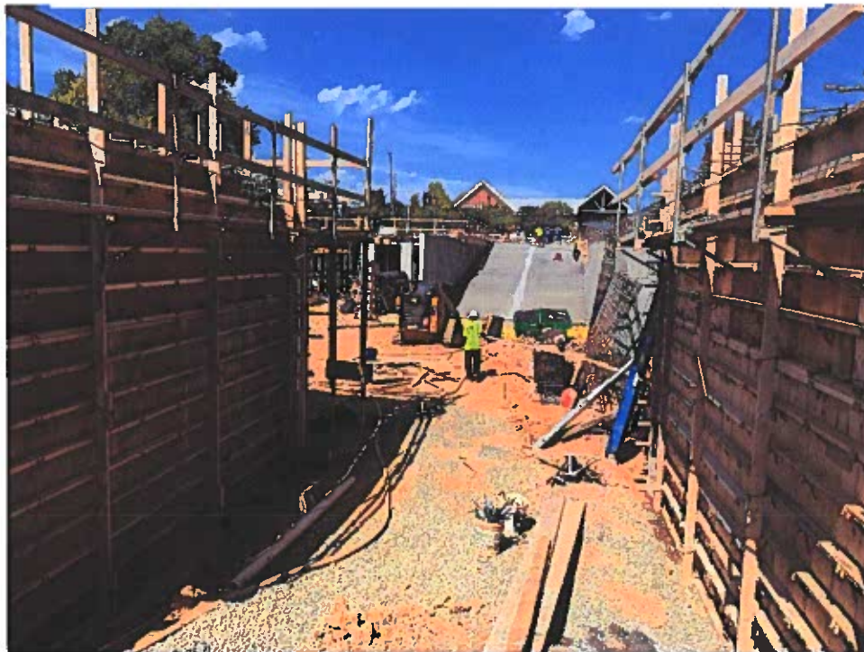
Figure 3 September 23, 2019; Looking north at garage ramp
