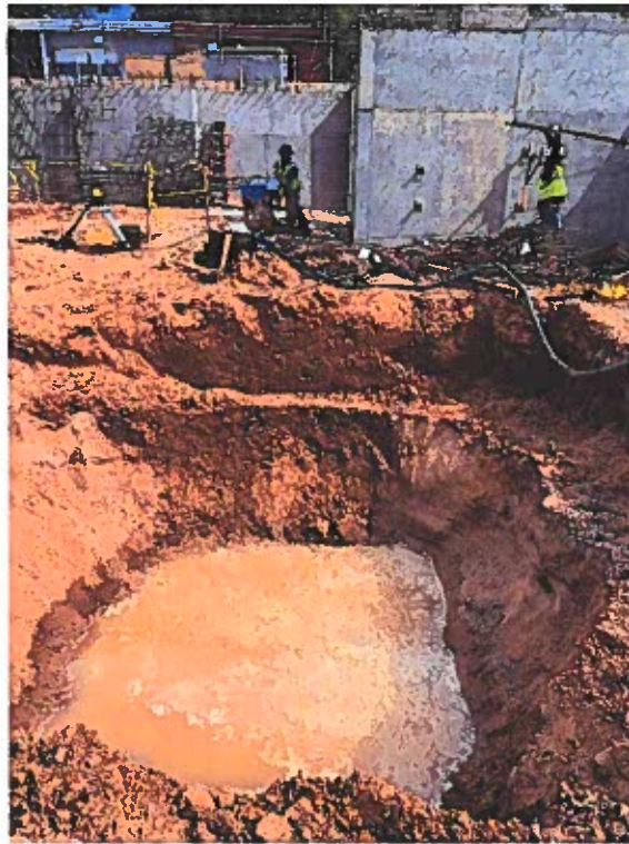
Figure 2 September 24, 2019: Water found at E11 footer excavation
