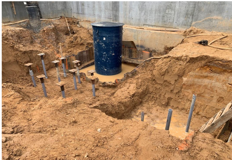
Figure 6 - October 25, 2019: View of sump pump and E11 & grease interceptor helicals
