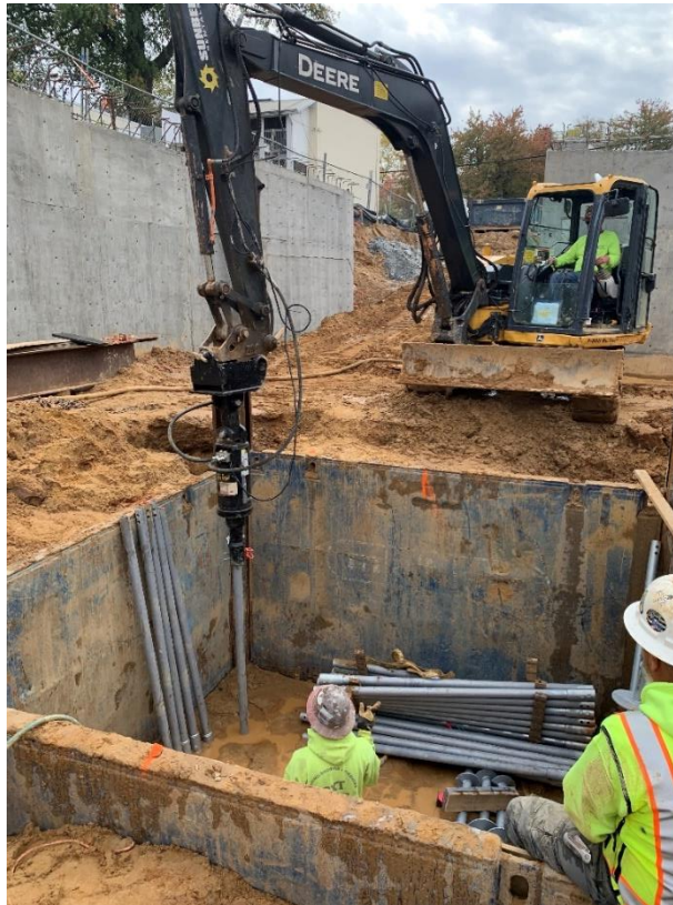
Figure 5 - October 25, 2019: View looking south of elevator pit helical install
