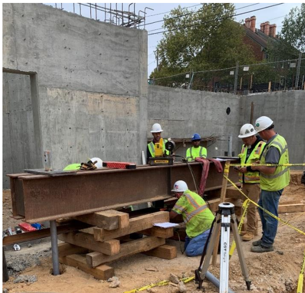
Figure 1 - October 8, 2019: Engineer running helical pile install test
