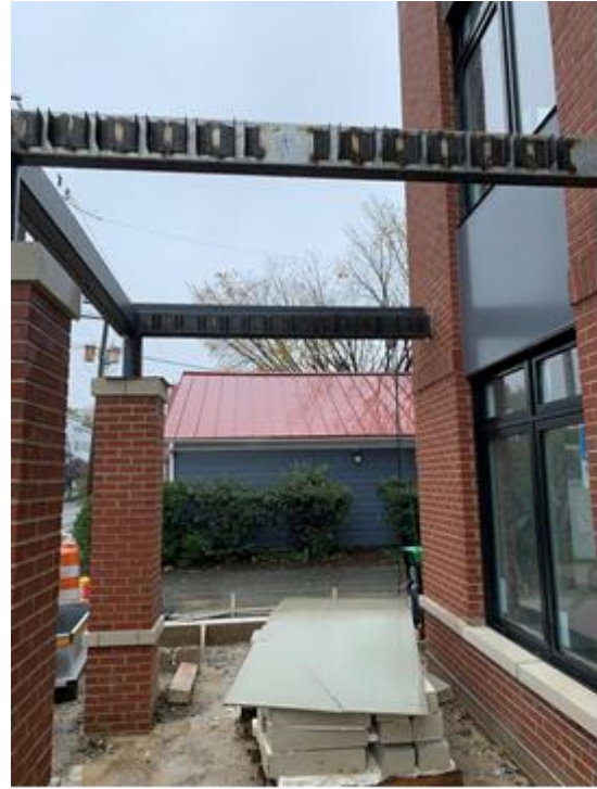
Figure 3 – Oct 30, 2020: Entrance canopies hangers welded
