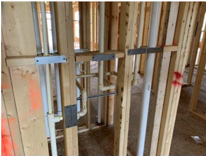
Figure 5 – April 28, 2020: Unit plumbing rough-in
