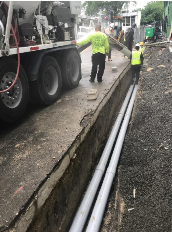
Figure 5 – May 28, 2020: Dry Utility Conduit in Alley
