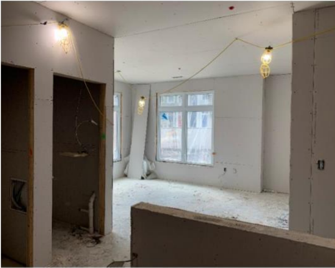
Figure 3 – June 26, 2020: Unit 102 with drywall hung
