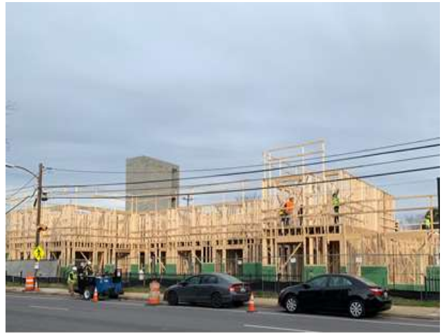
Figure 4 – January 30, 2020: Looking northeast at the first and second floor framing
