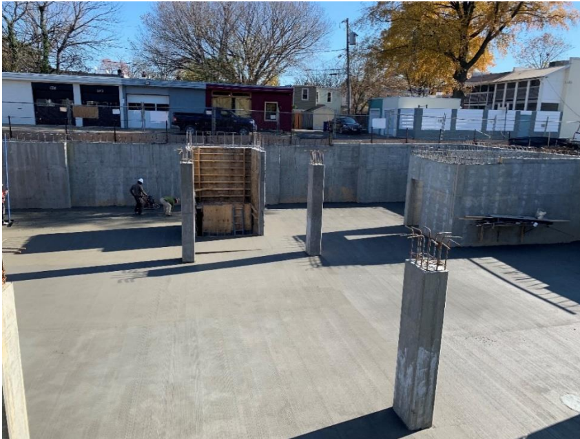
Figure 3 – November 25, 2019: Looking east at the newly poured garage slab
