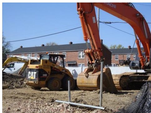
Construction at Old Town Commons
